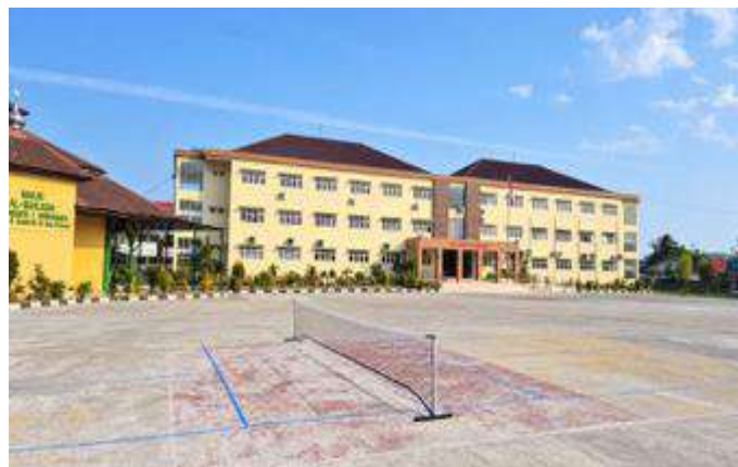
Figure 3. The condition of the pickleball court after it is finished
